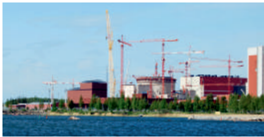
Olkiluoto 3 under construction in 2009. It is the first EPR design, but problems with workmanship and supervision have created costly delays which led to an inquiry by the Finnish nuclear regulator STUK. In December 2012, Areva estimated that the full cost of building the reactor will be about 8.5 billion, or almost three times the original delivery price of 3 billion.
