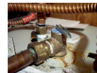
Temperature and Pressure safety valve on a water heater.
