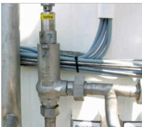
An oxygen safety relief valve
