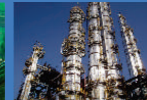
Butadiene Extraction Plant Reliance Industries Limited
