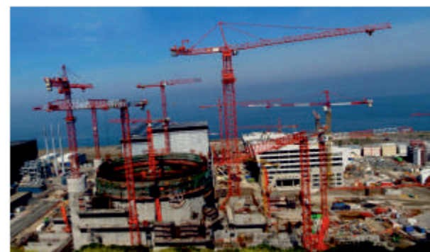
EDF has said its third-generation EPR Flamanville 3 project (seen here in 2010) will be delayed until 2018, due to "both structural and economic reasons," and the project's total cost has climbed to EUR 11 billion in 2012. Similarly, the cost of the EPR being built at Olkiluoto, Finland, has escalated dramatically, and the project is well behind schedule. The initial low cost forecasts for these megaprojects exhibited "optimism bias".
