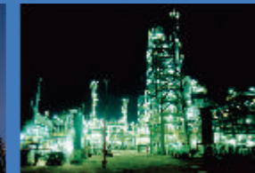
Refinery Expansion Project Mangalore Refinery & Petrochemicals Ltd.
